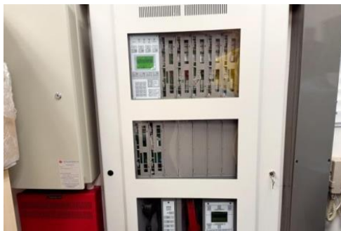
Fire Alarm Control Panel
